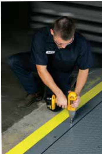
Engineer during installation at site
